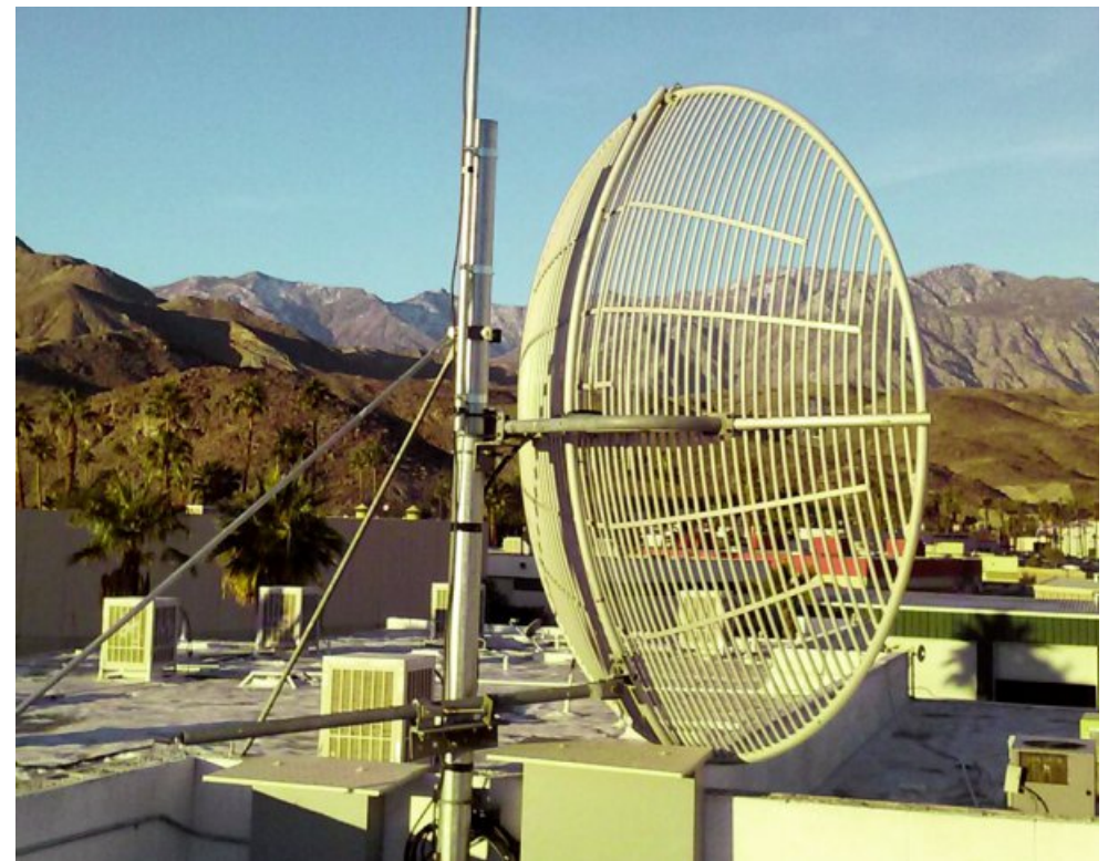
Fig-5 Feed mounted on a 8 ft. grid dish
