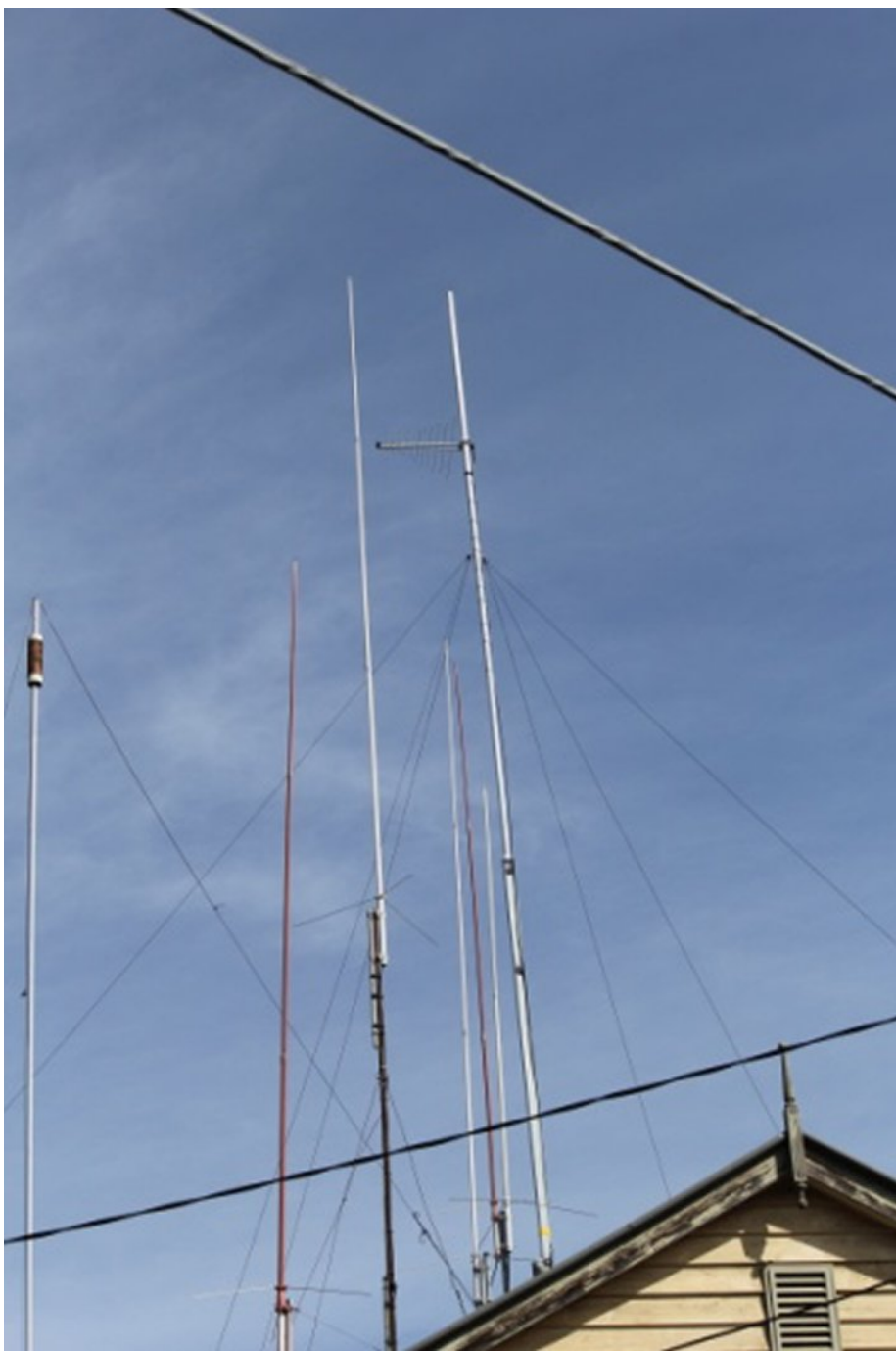
Six black guy ropes can be seen attached just under the log periodic TV yagi beam.
