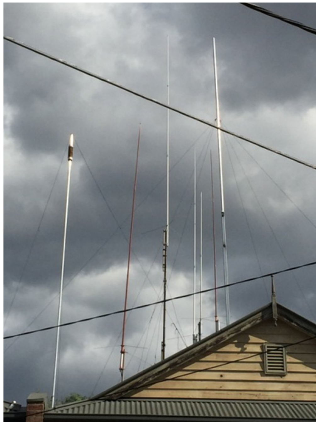
The new mast seen without anything on it on left and just a TV antenna attached on the right as a wind load test before adding the rest.
