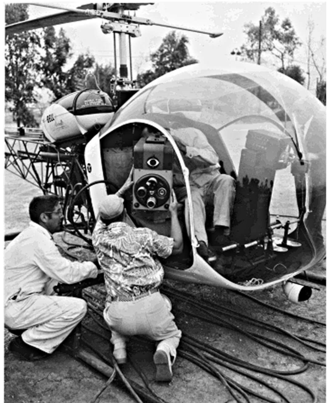
In the early or mid 1950's, CBS Engineers place a RCA-TK-30 Camera in a Helicopter
