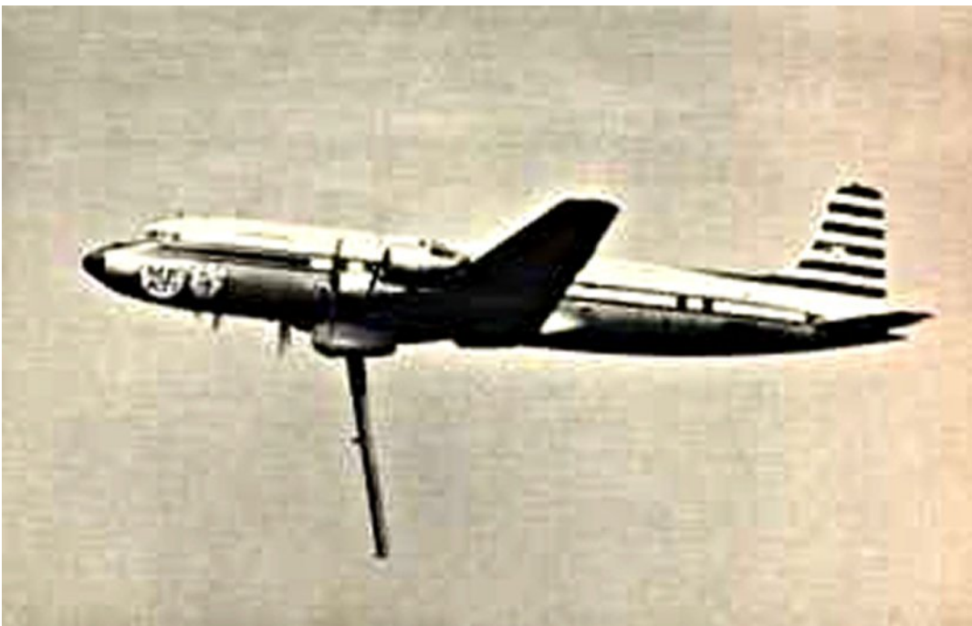
DC6 with a forty-foot gyroscopically stabilized antenna mast
