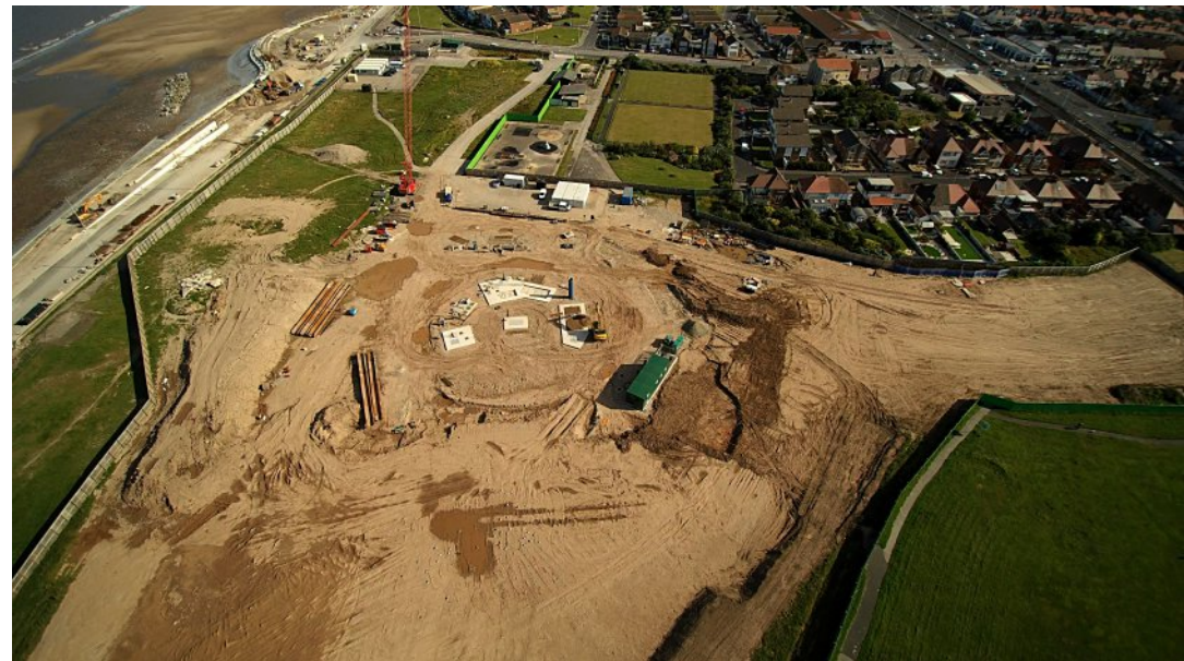
Anchorsholme park in early July
