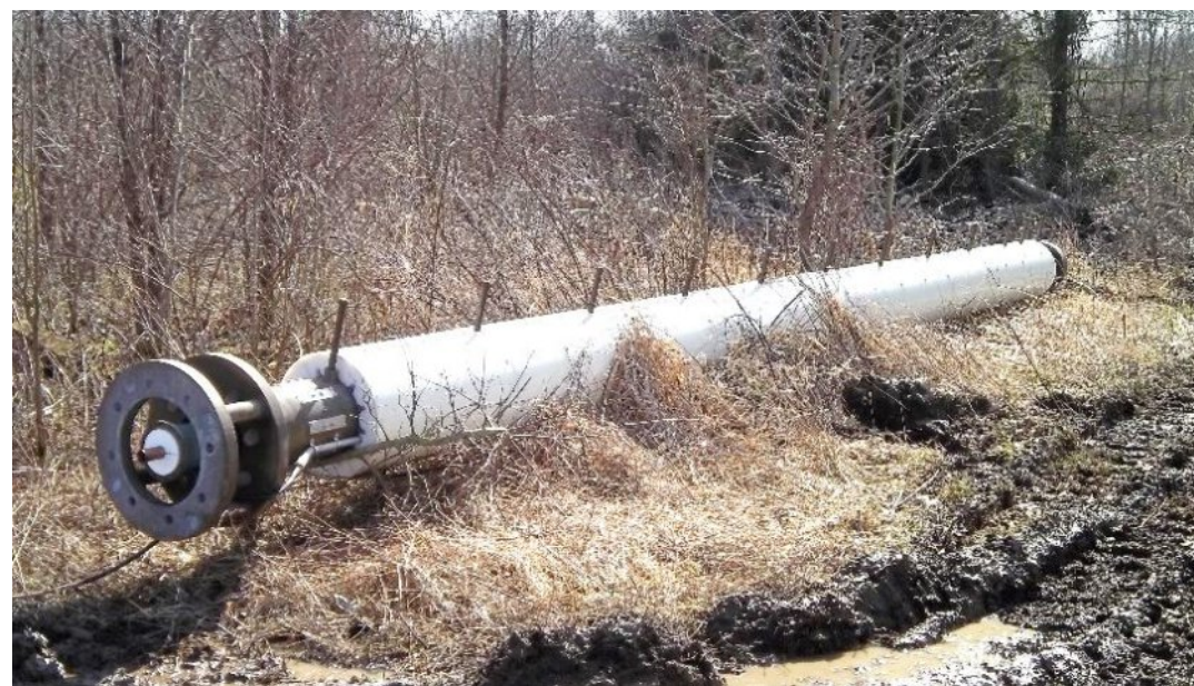
The removed old antenna. Notice the climbing spikes.
